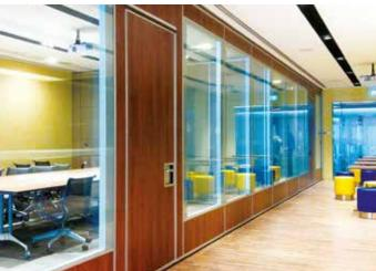
Acoustic operable glasswall maintains the aesthetic appeal of glass while providing acoustic separation to STC 44. Acoustic operable glasswalls are available as single and paired panels only. They consist of glass surrounded with an aluminum frame that is nominal 83mm thick. Each panel has a 25mm clearance bottom retractable seal that exerts downward force. The standard aluminum frame finish is clear anodized but it may also be ordered powder coated or custom anodized.
